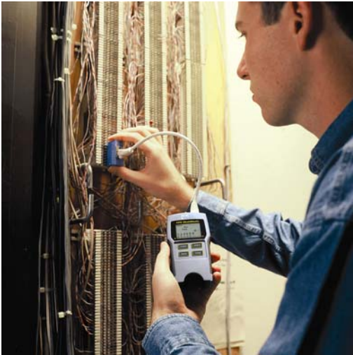
Picture 1: VDV MultiMedia Cable Testing
