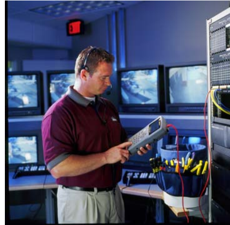
Picture 3: LAN cable certification with LANTEK
